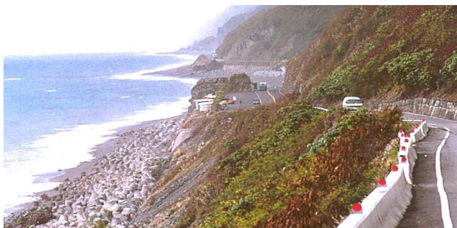
Fig. 4. Revetment with armor units for toe protection at Taimalicoast, Taitung county
