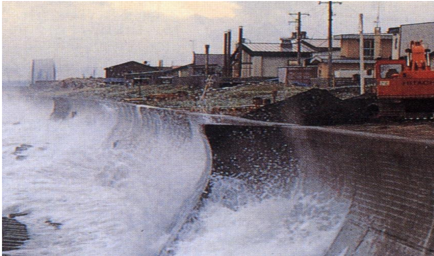
Fig. 15-16. The seawall and revetment built at south coast of Taiwan(Conventional countermeasures against beach erosion)
