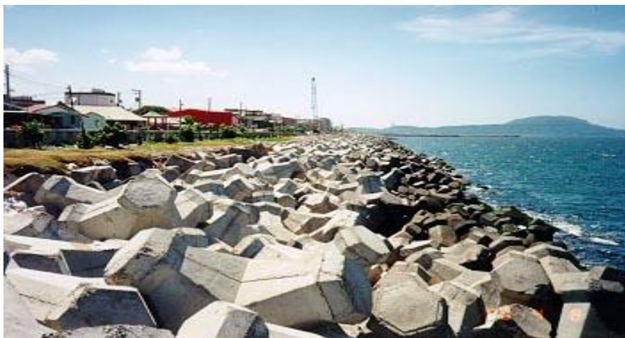
Fig. 3. Seawall with armor units in the fronting faces at Ketzeliacoast, Kaohsiung county.
