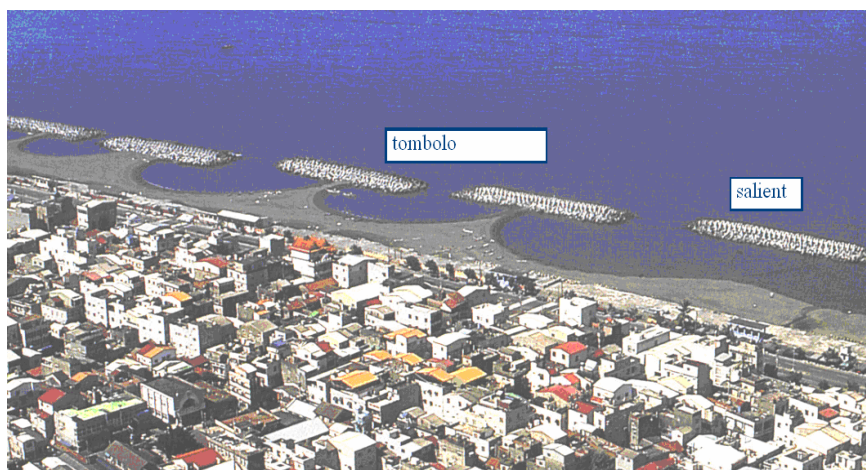
Fig. 16. Effectives of detached breakwaters at Cheding coast, Kaohsiung County
