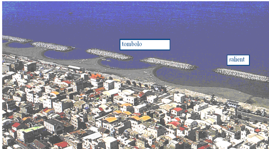
Fig. 2. Detached breakwater at Cheding coast, Kaohsiung county.
