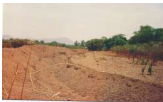
Plate 1: Trench was dug on the left bar to shift the channel
