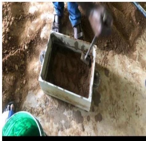
Figure 1. Ramming process with the use of flat rammer
